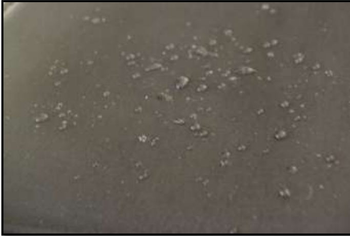
Figure 7: Water Repellant after Sealing.
